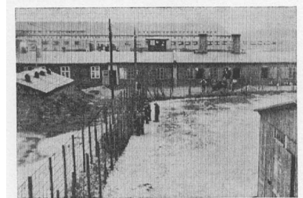
Flak School from Guard Tower
